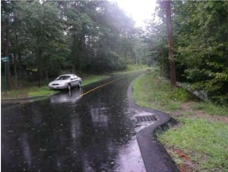
**The asphalt berm and infiltration basin installed by Town of Mashpee capturing all stormwater runoff from Timberlane Drive and Lantern Lane on August 29, 2009.**
