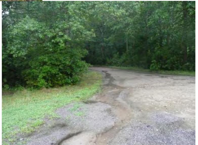
**Stormwater runoff flowing from Town landing access road and parking lot directly into Santuit Pond (WW-1) on August 29, 2009.**
