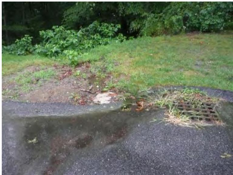
**Stormwater runoff not all being captured by infiltration basin on Beachwood Point Drive (WW-4) and flowing toward Santuit Pond on August 29, 2009.**
