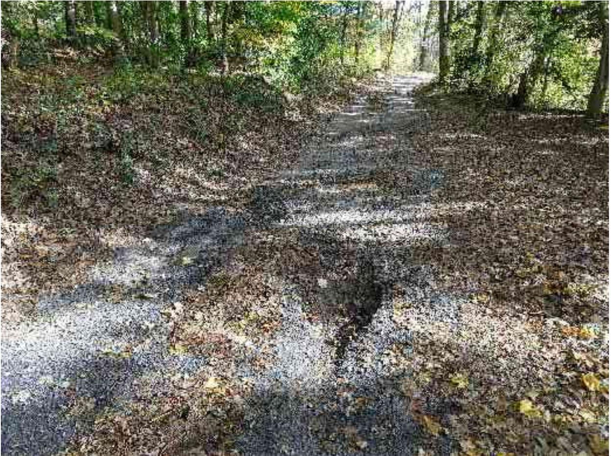
Photo 34) Town Landing (erosion along side of access road)
