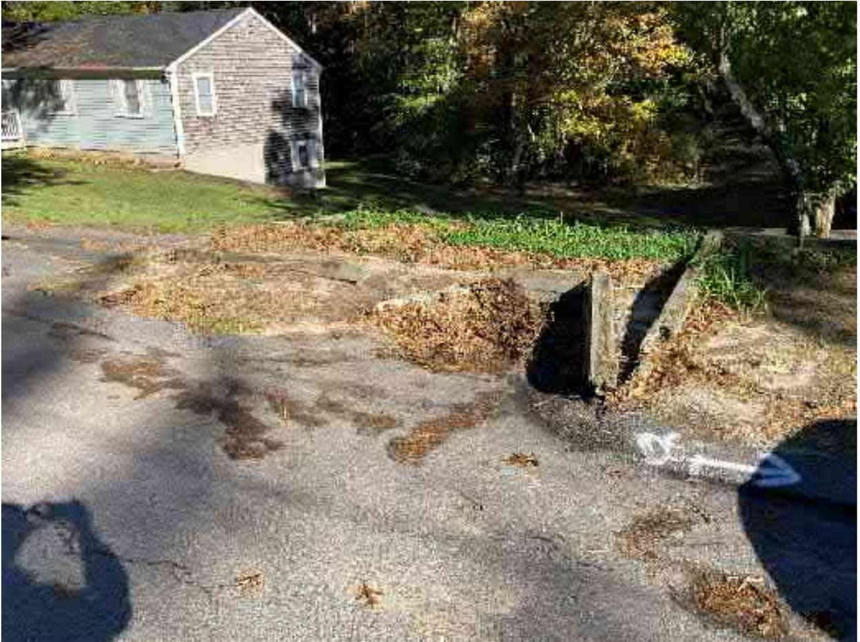
Photo 8) 5 Autumn Drive (flow path of stormwater bypass down driveway)
