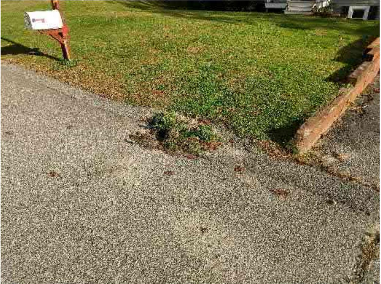
Photo 14) Leamington Lane/Cotuit Road Intersection (clogged catch basin and heavy debris on Leamington)
