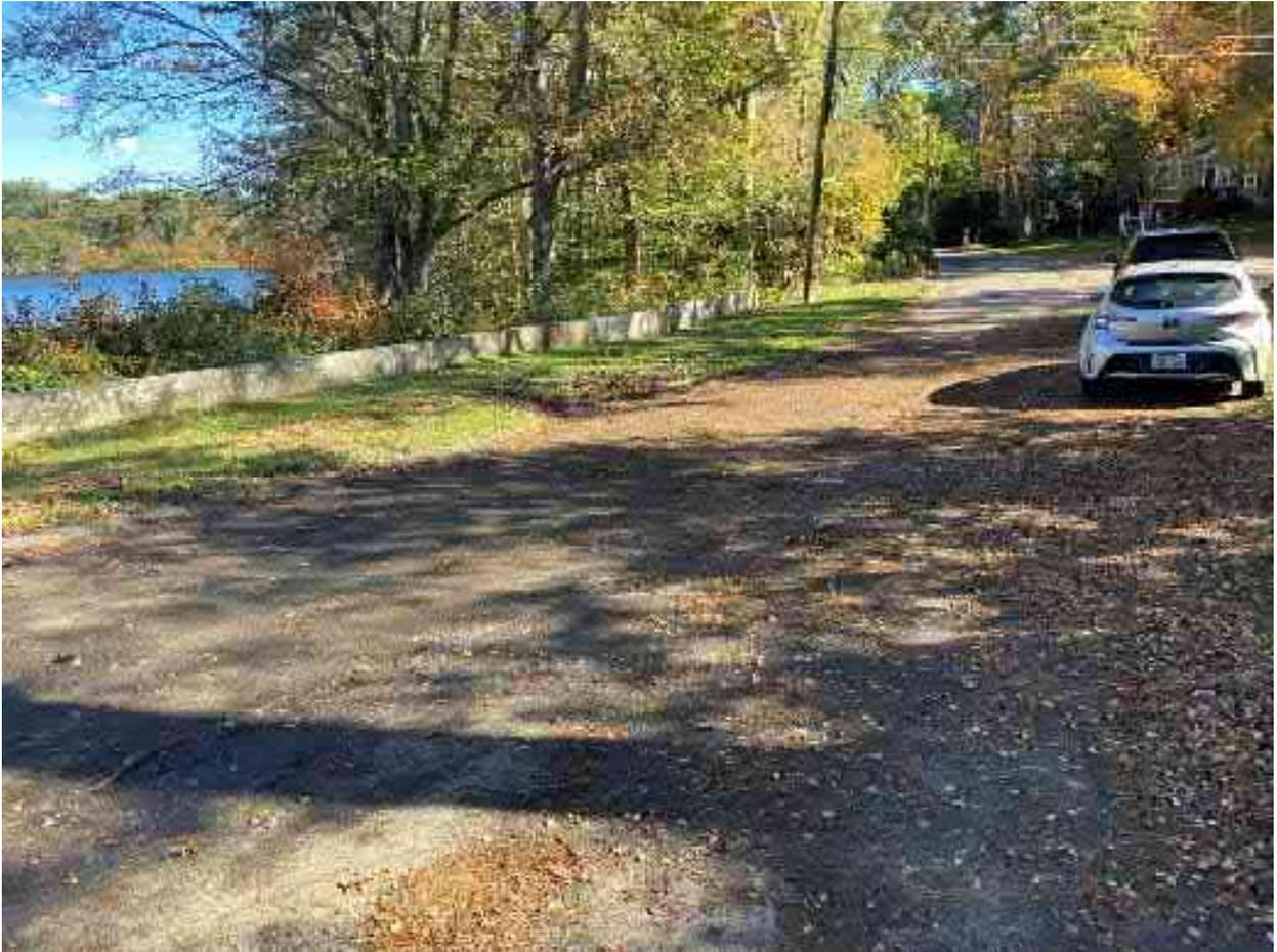
Photo 44) Timberlane Drive Upgradient of Town Landing Access Road (stormwater bypass of catch basin)
