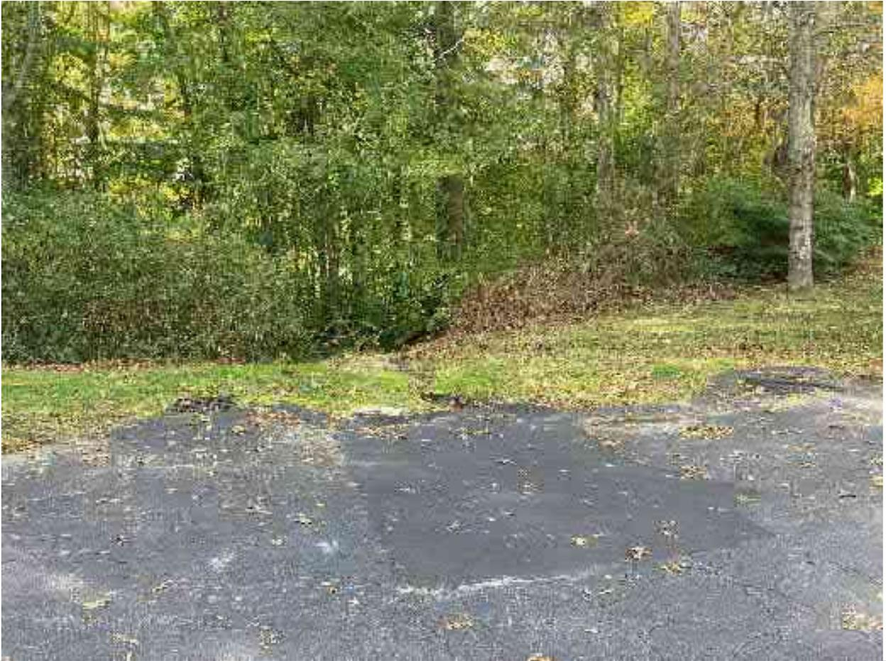
Photo 52) Beechwood Point/Santuit Pond Way (erosion gully to wetlands from edge of parking lot)
