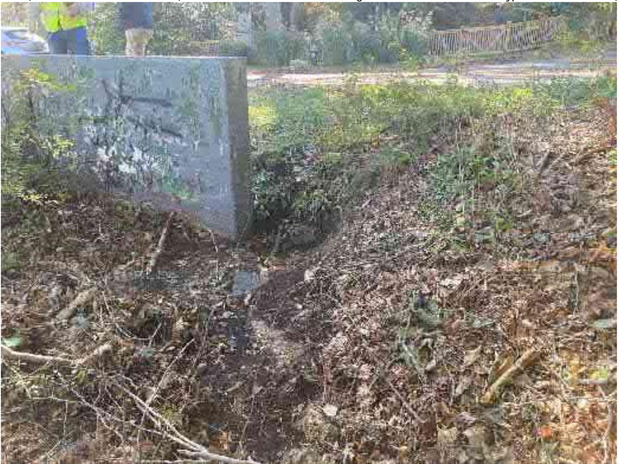
Photo 42) Timberlane Drive (rutting and overland flow path towards pond)
