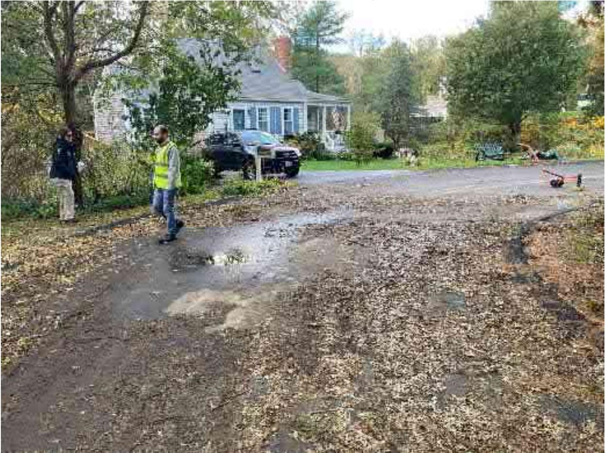
Photo 10) Deerfoot Circle Cul-de-Sac (stormwater bypass of catch basin)
