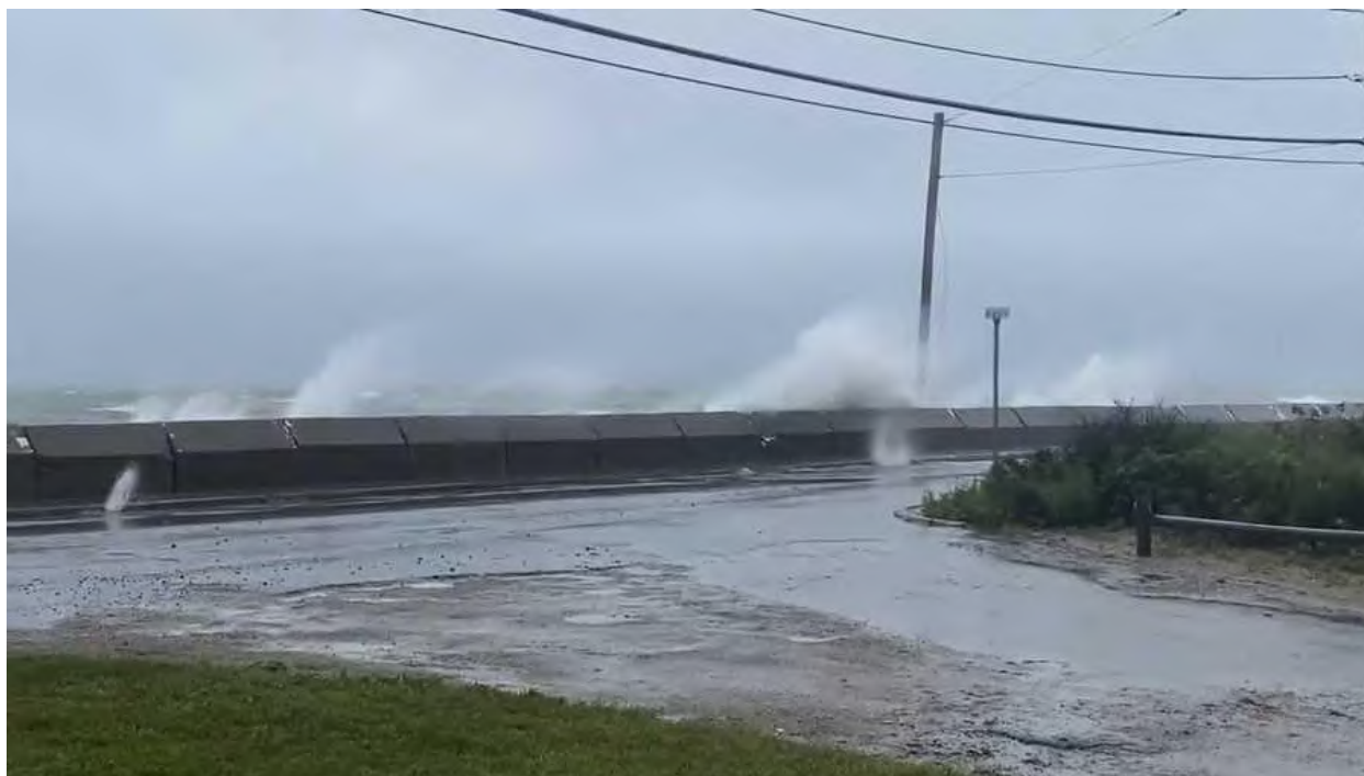
Figure 3-13. Large waves overtopping the seawall along Menauhant Road during Tropical Storm Henri on August 22, 2021.
