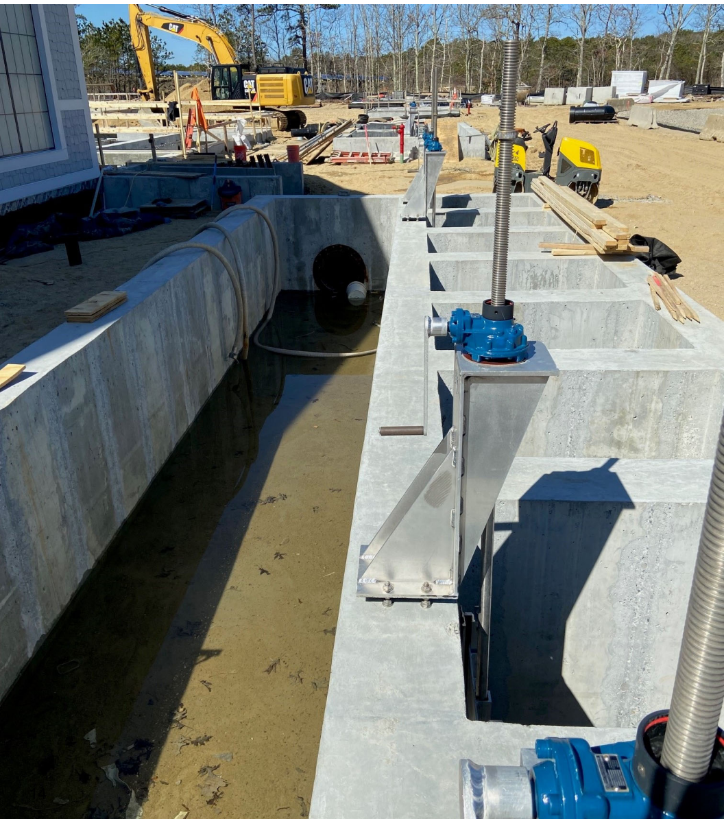
Influent Pump Station Wet Well Distribution Boxes
