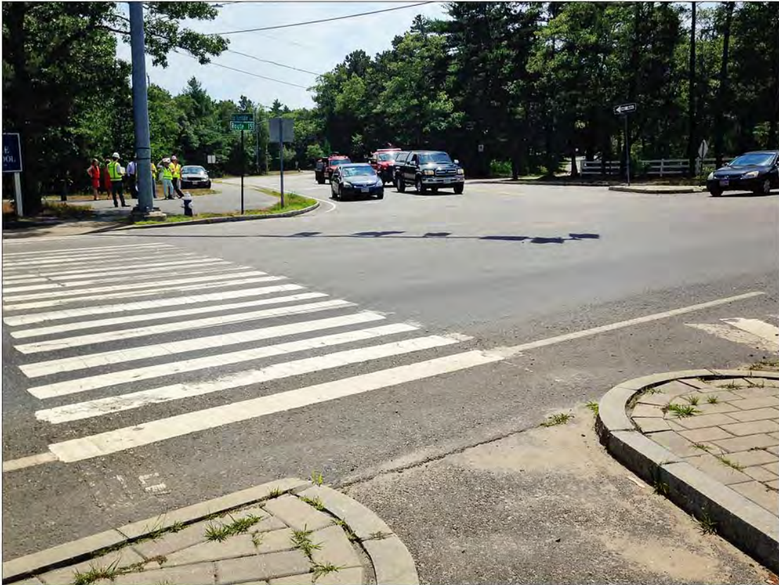
Southbound view from the pedestrian island looking onto traffic stopped on Old Barnstable Road.
