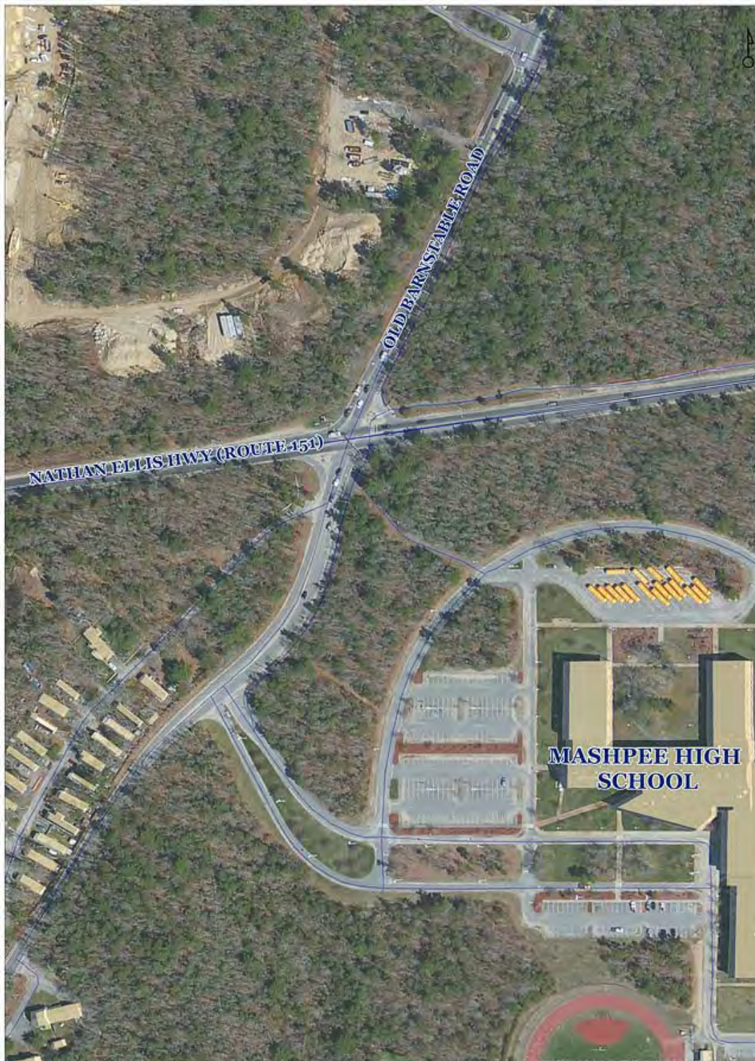
Figure 2. Nathan Ellis highway (Route 151) at Old Barnstable Road intersection.
