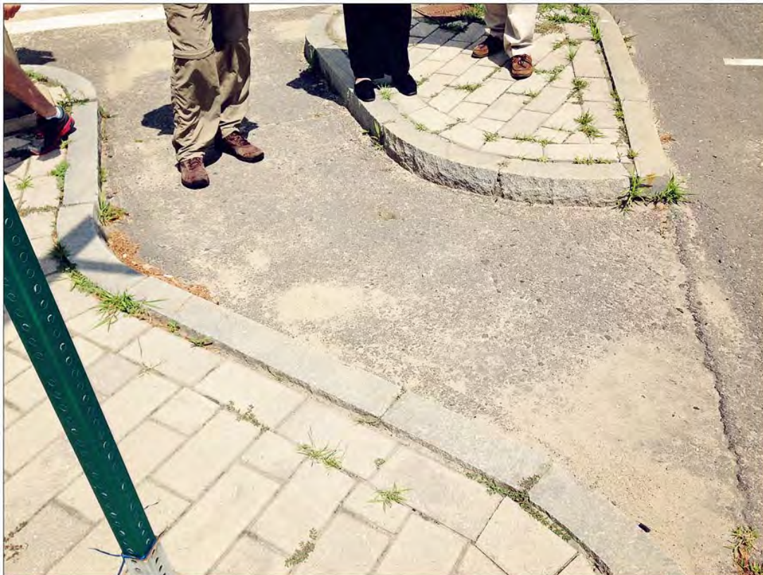
Pedestrian accommodation island in the north east quadrant of the Old Barnstable Road/Route 151 intersection.
