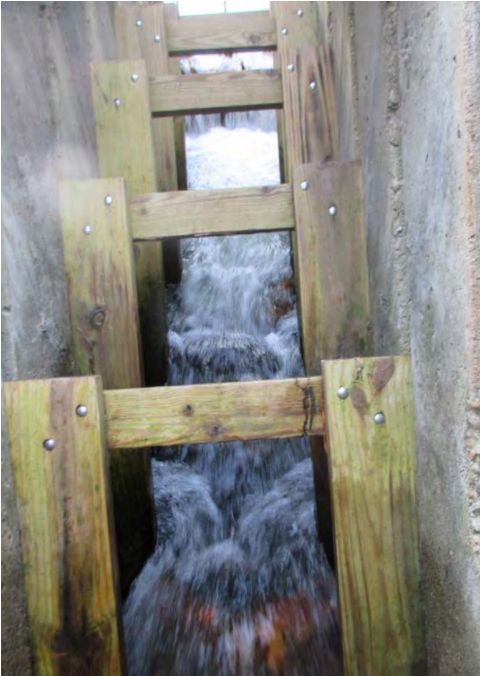
View of existing turbulent - high velocity - fish ladder
