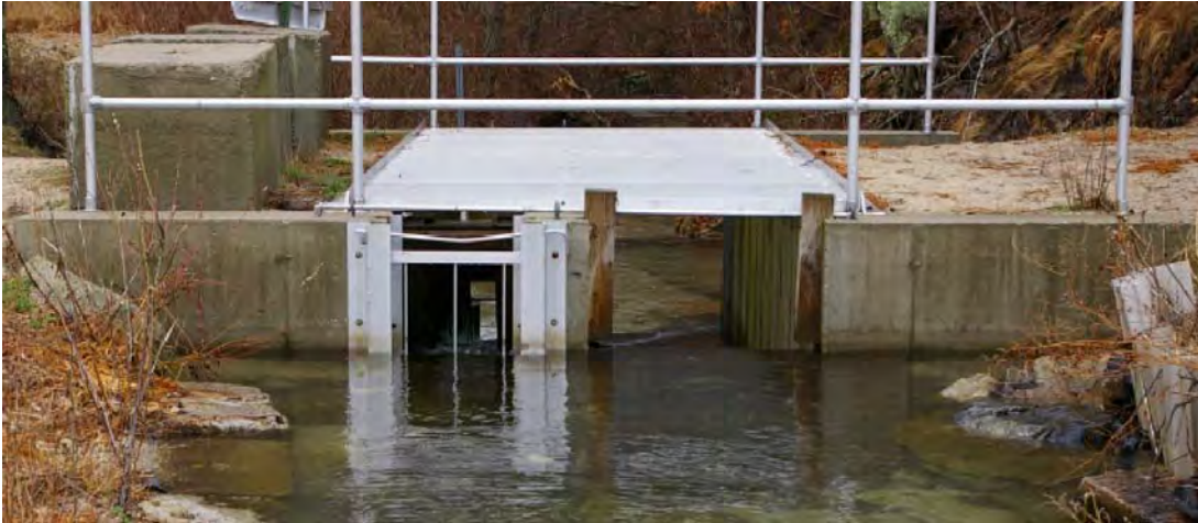
Photograph of outlet weirs (looking down stream)
