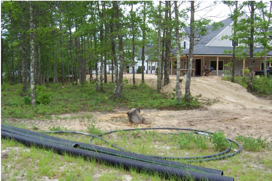
Cape Cod Coffee from Evergreen Circle close to Route 130. Sloped fill in front of building does not exceed plan limits. Fill to right and in foreground is part of area that was to remain natural.
