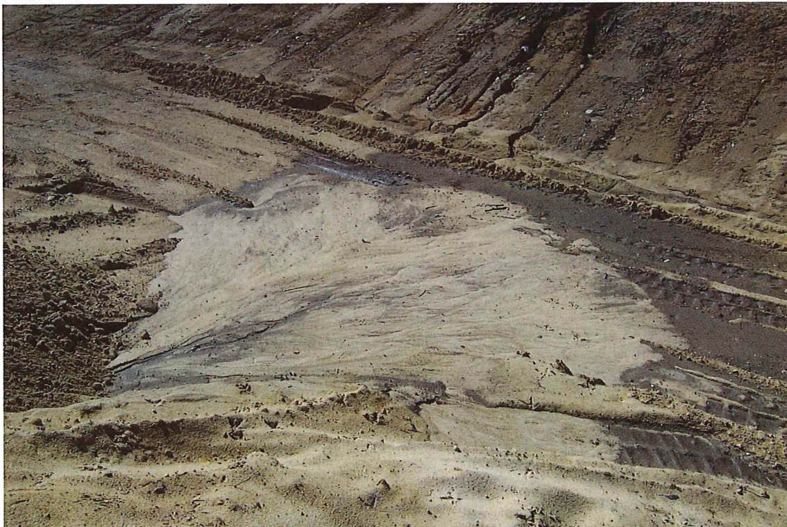
Midpoint of Drainage Area on Carriage Drive, Erosion from Edge of Pavement
