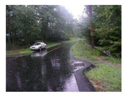
The asphalt berm and infiltration basin installed by Town of Mashpee capturing all stormwater runoff from Timberlane Drive and Lantern Lane on August 29, 2009.
