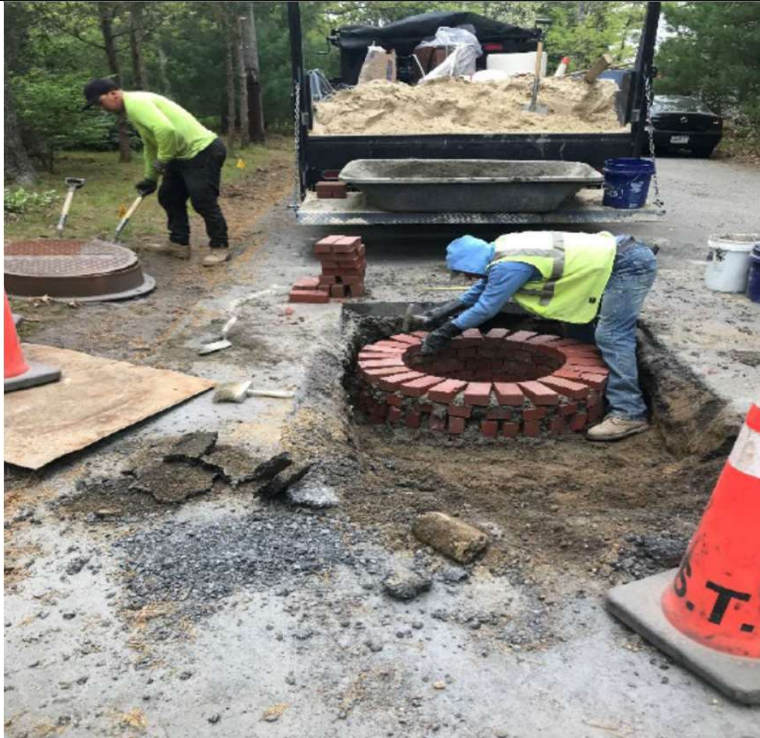
Installation of Manhole Frame and Cover on Shipwreck Drive
