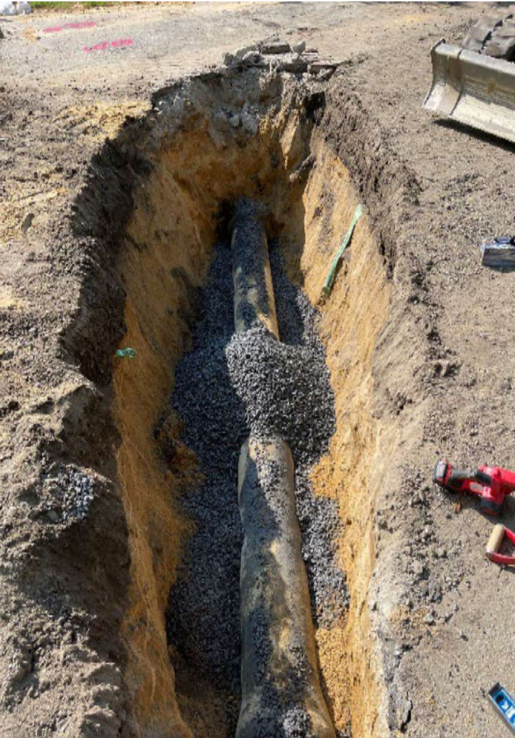
Reinstallation of Drain Pipe
