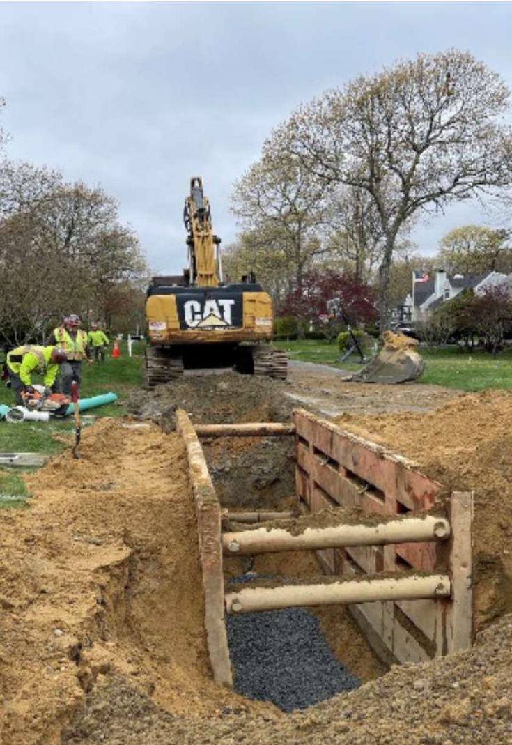
Installation of Gravity Sewer
