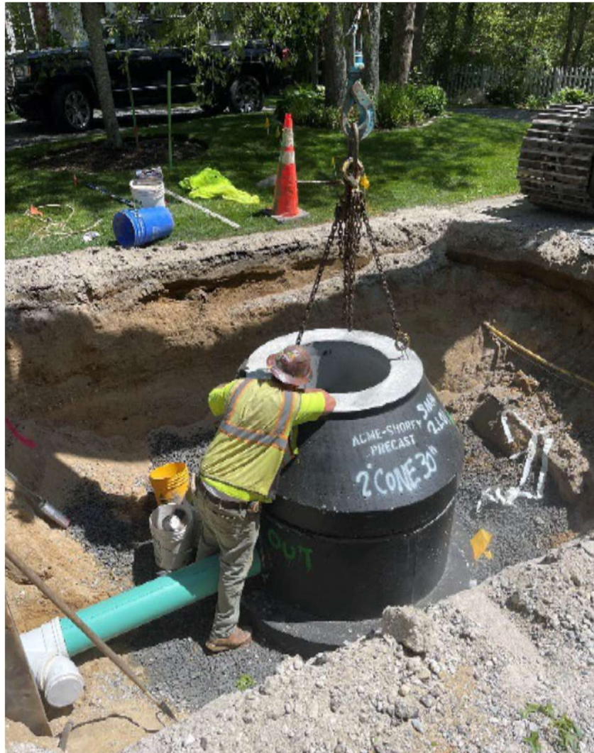
Installation of Manhole
