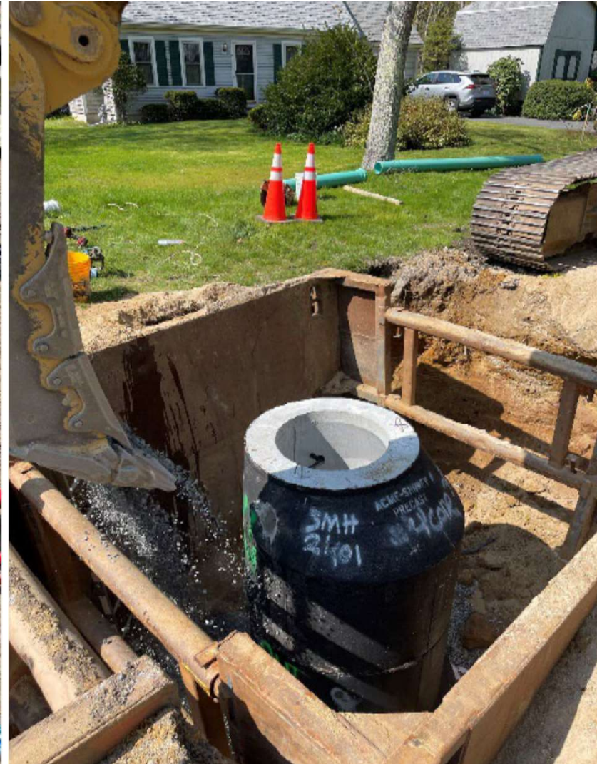
Installation of Manhole
