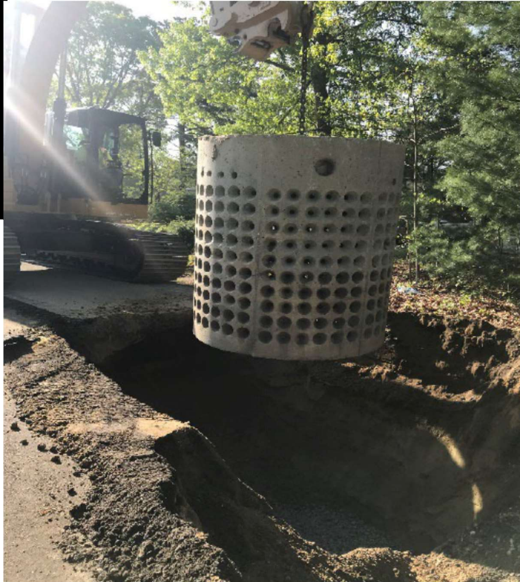
Installation of Leaching Pit on Ships Anchor
